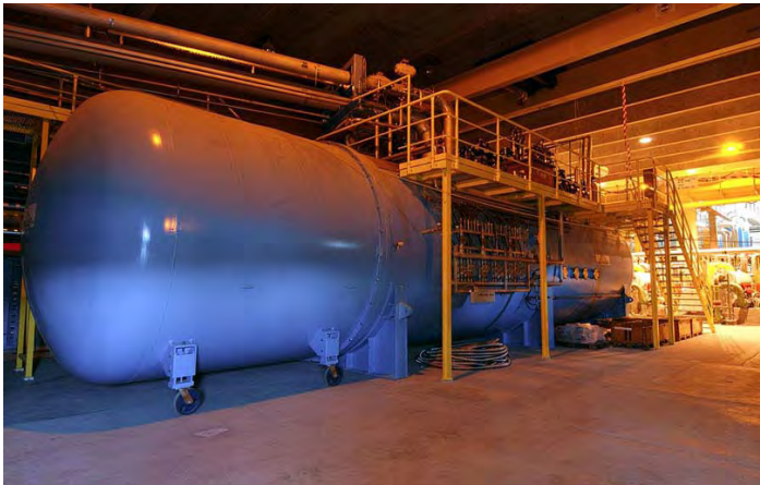
A helium refrigerator for the LHC.
