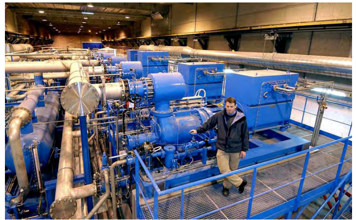
A helium compression station for the LHC.
