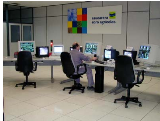
Fig. 2. Plant operator in a control room
