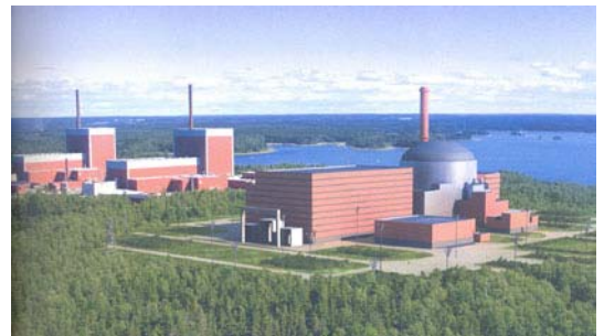
C. Nuclear de Olkiluoto 3 PWR-Areva 1.650 MWe
