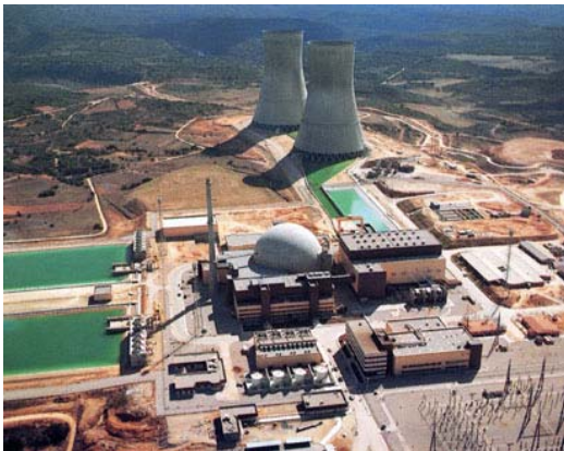
Trillo NPP PWR-KWU 1050 MWe
